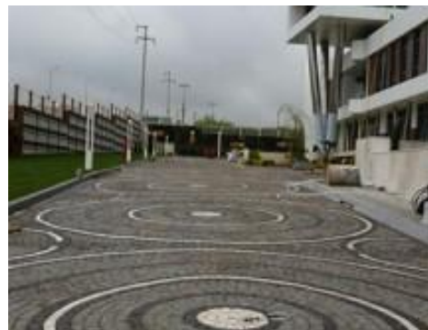
f. traffic facility construction
