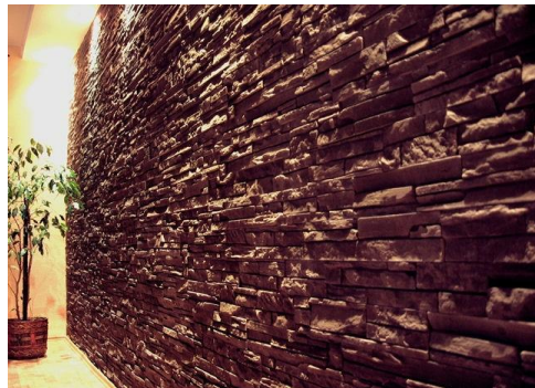
c. wall cladding with basalt
