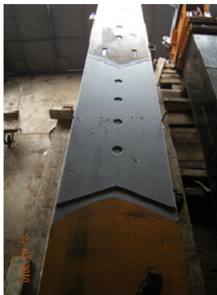
Figure 6: Appearance of steel construction of auto crane after repair
