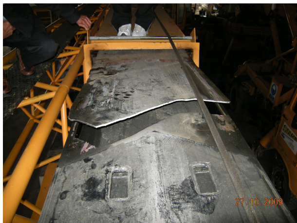
Figure 1 Crack of telescopic arm of vehicle-mounted crane
