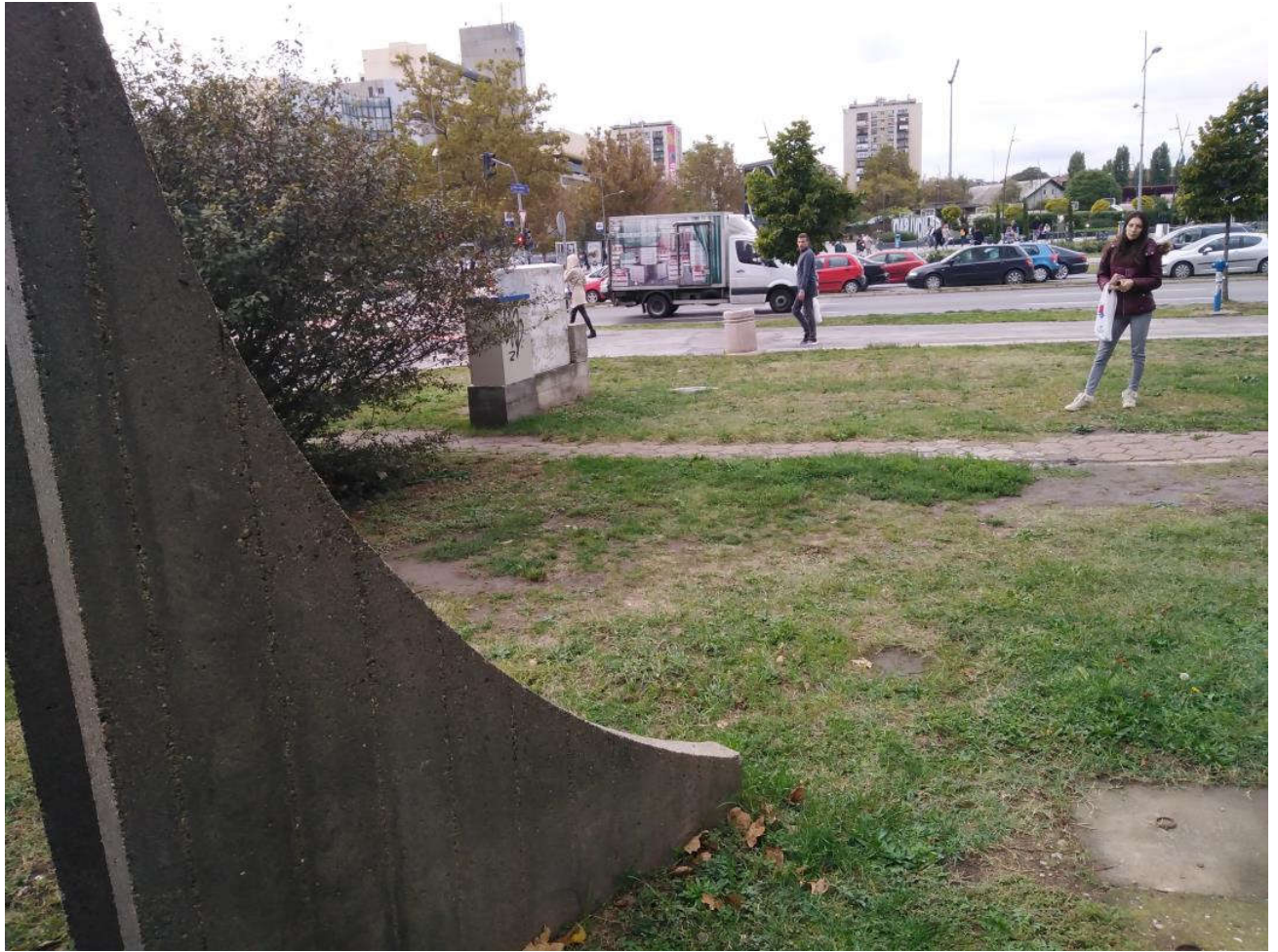
Figure 9. Lower right hand corner shows the shaft now covered with a RC slab. Photo taken in 2022.
