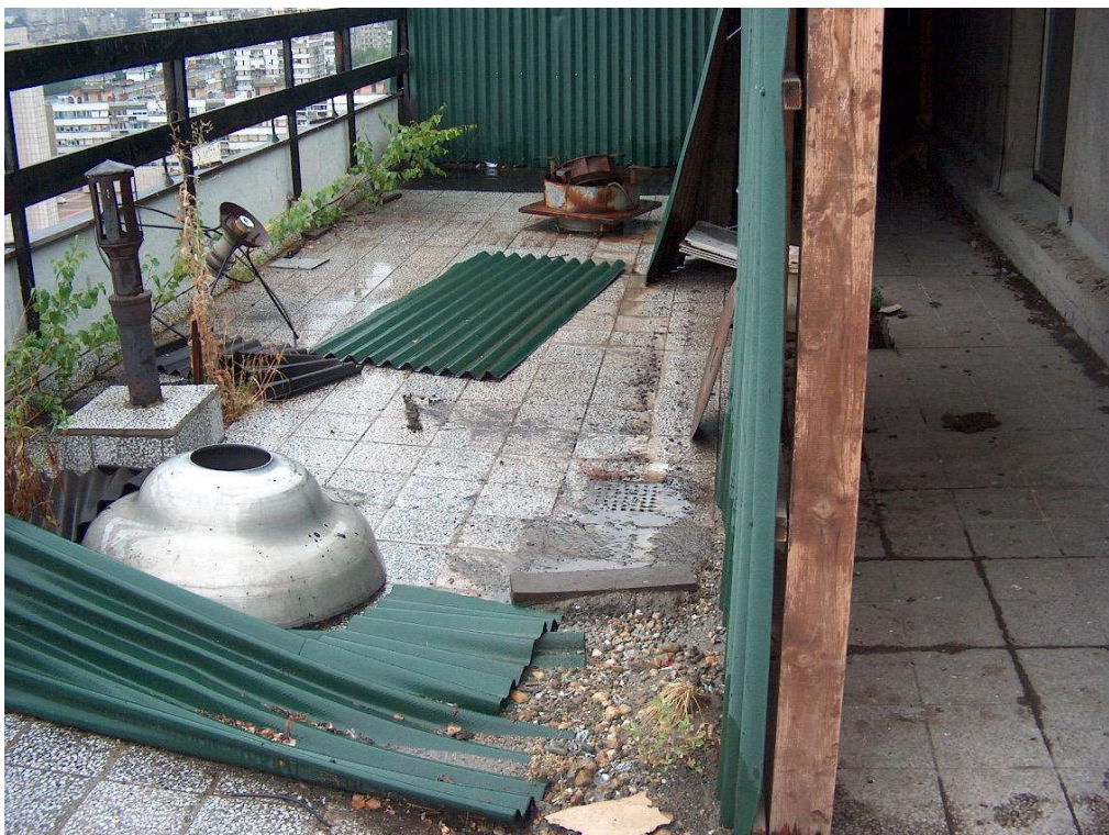
Figure 8. A view of a smaller rooftop terrace and a drain. July 2004.
