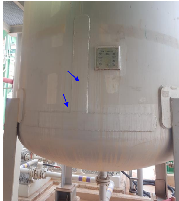
Figure 3. Installed welded patches.
