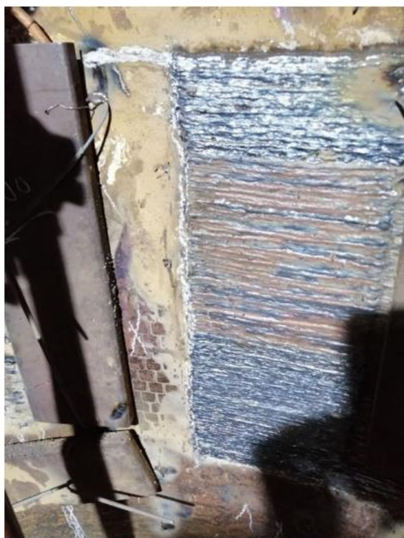
Figure 2. Repair welding of connecting vessel mantle thinned walls.
