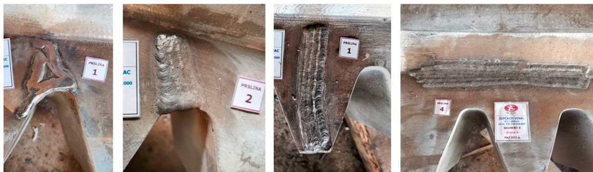
Fig. 4. Filled grooves on gear segments.
