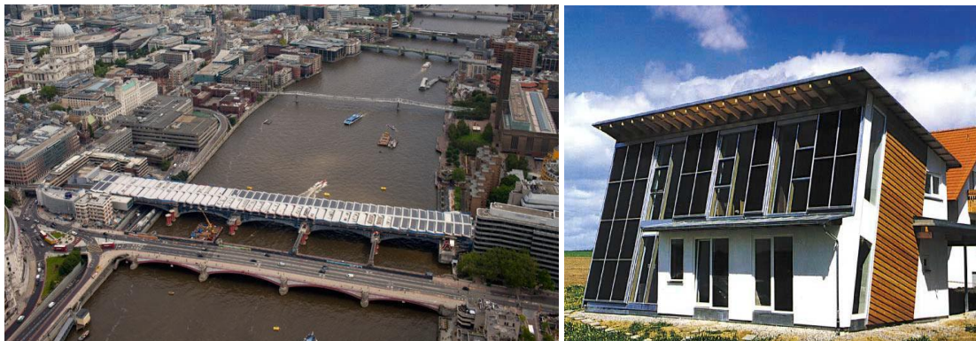
Figure 3. Solar bridge in London and solar-roof and facade 24 m 2 in Germany [17]
