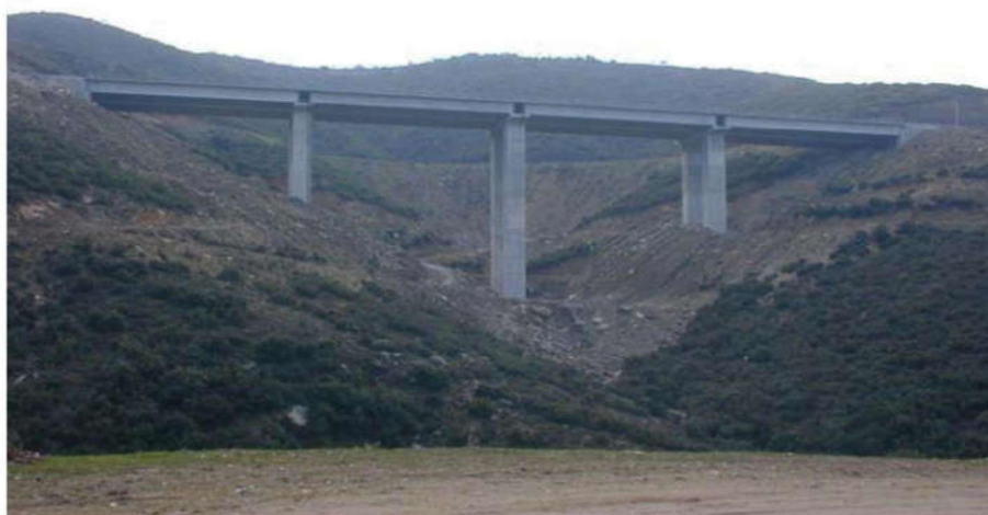
Fig. 1: The Kavala bridge on Egnatia Motorway, East Macedonia.
