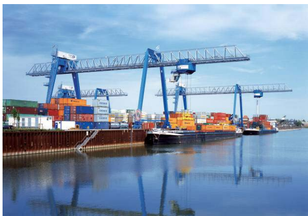
Figure 13. Quayside container crane with 3D truss girder
