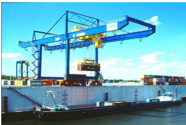
Figure 12. Quayside container crane with box sections
