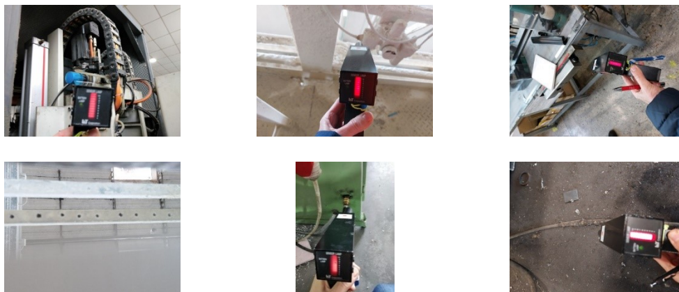
Figure 2 Leaks detected during energy audits [2]
