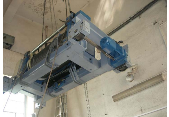
Figure 12: Installation of the equipment
