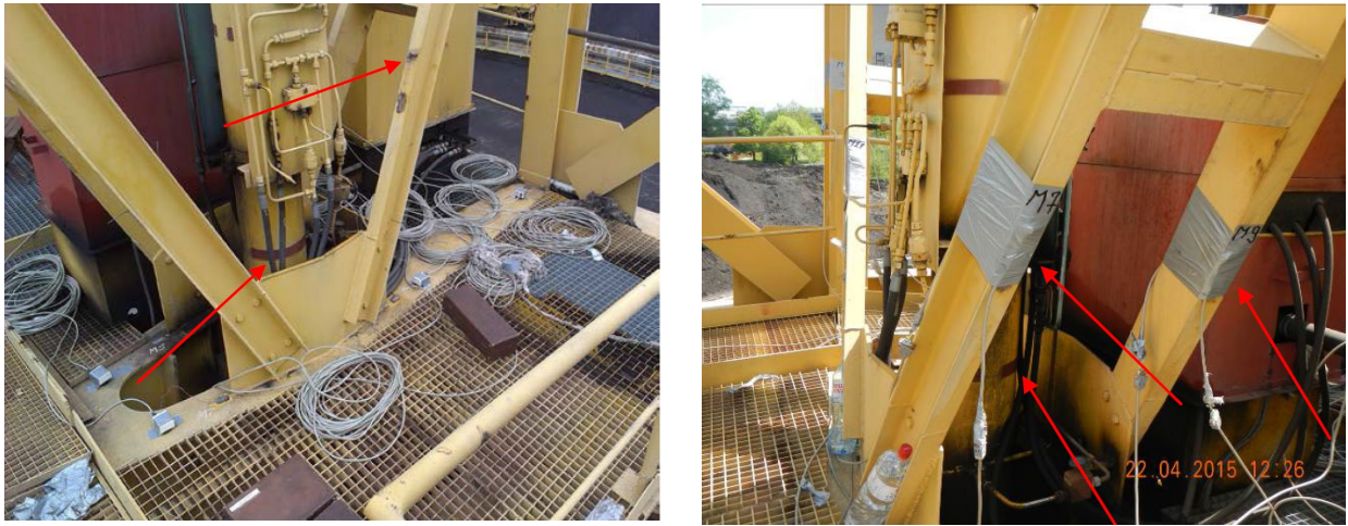
a) Measurement locations right of the support structure
