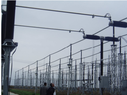
Fig. 6. Improved dynamic (and static) rigidity of the system by transforming fixed support into clamp
