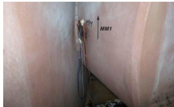
Figure 5 The strain gauge in measuring spot MM
