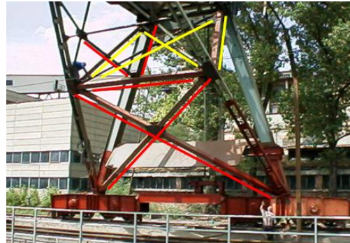
Fig. 16. Redesigned bracing truss
