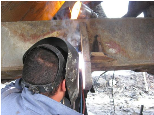
Fig. 10. Welding of the redesigned rear support eye
