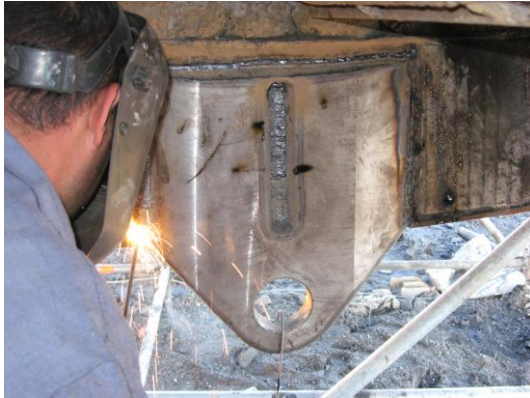
Fig. 9. Welding of the redesigned front support eye
