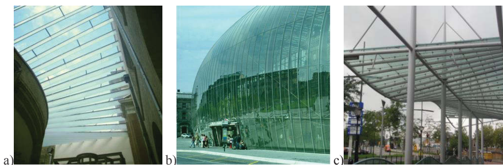
Figure 4 – Cold bent glass applications (by assembling): a) Victoria & Albert Museum, London; b) Train Station TGV, Strasbourg; c) Bus Station – Zuidpoort, Delft
