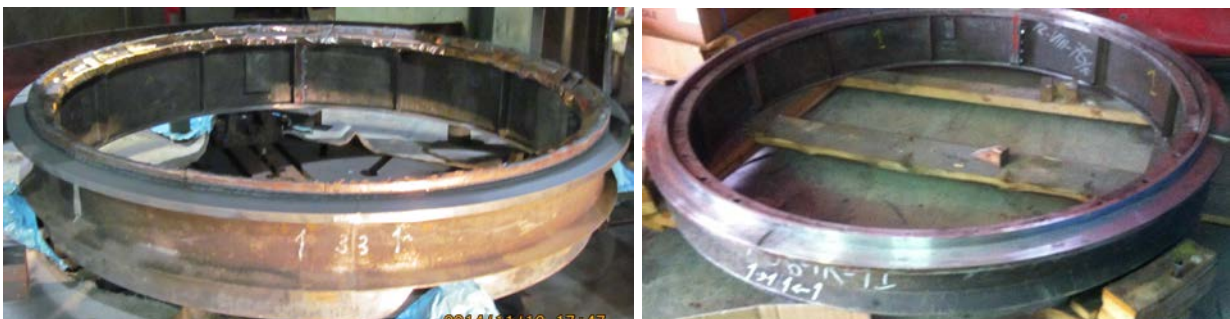
a) Appearance of the flange before the repair b) Appearance of the flange after the repair by cold metallization
