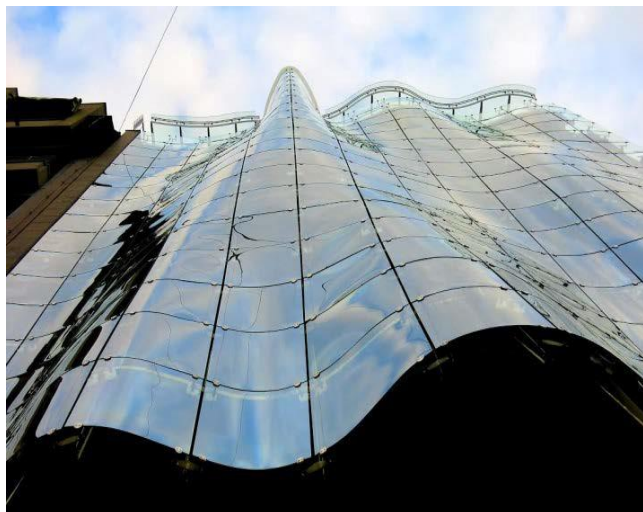
Figure 1. Glass facade of residential building 'Infinity'.
