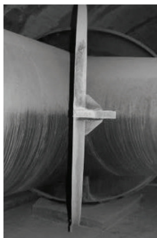
a) Proper mutual position of the collar and the anchor
