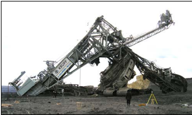
Figure 3: BWE Sch Rs 1760 after the collapse
