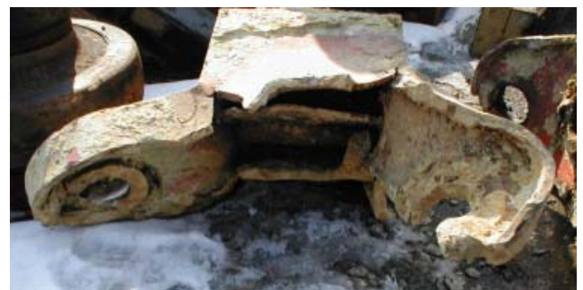
Figure 2: Typical failure of the TWB structure
