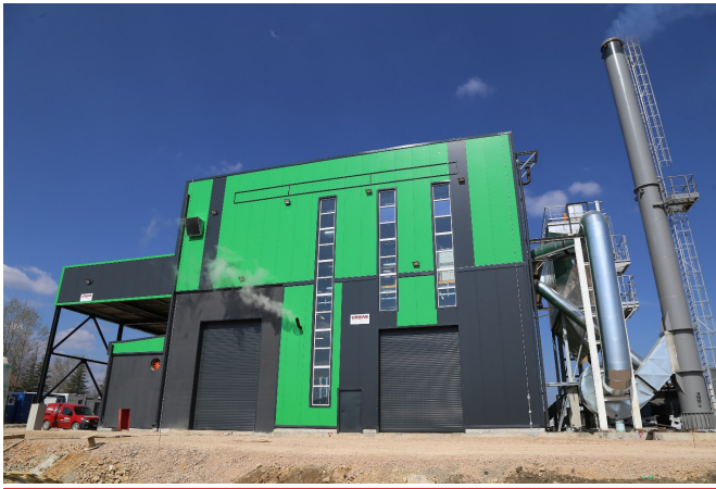
Figure 2: BEP's CHP plant Boljevac
