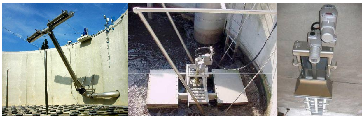
Fig. 1. From left: Pipe decanter, decanter-floating, wall-mounted decanter
