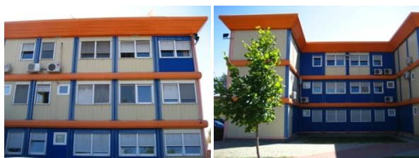
Figure 2b. Intermodal steel building units in Novi Sad, Serbia for office purposes
