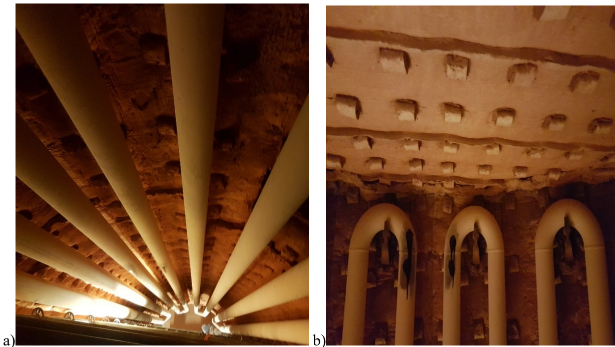
Fig. 2. Visual inspection showed that pipes are in good condition
