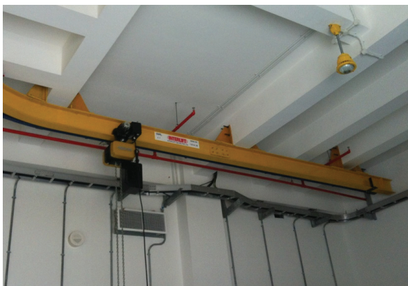
Figure 1. Runway beam for hoist with trolley
