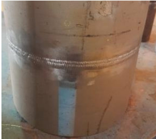
Figure 3. Butt weld joint SS-SS.
