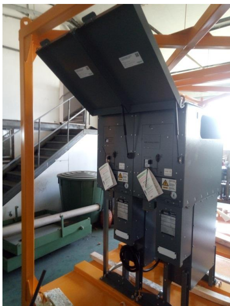
Figure 12. Equipment being installed on the base.
