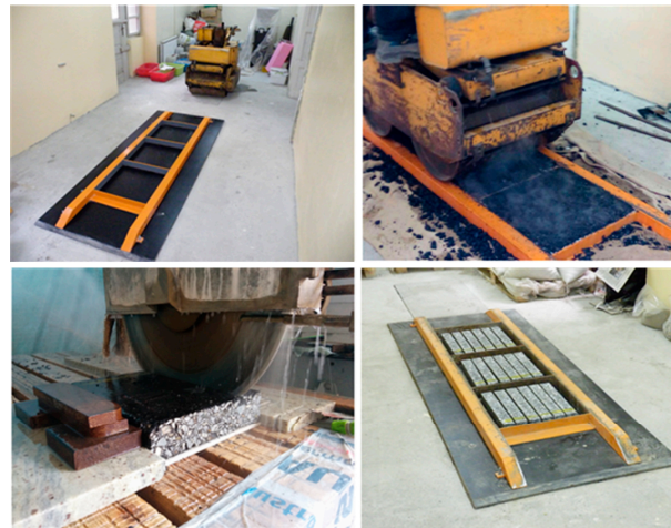
Figure 4. Asphalt mixture laying and compaction.
