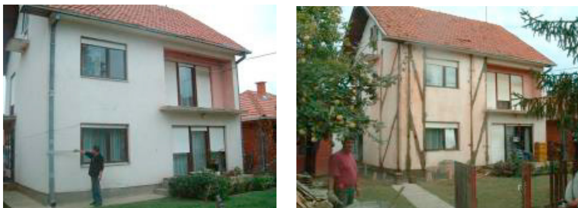
Fig. 2. (a) 3D House before retrofit (; (b) House after retrofit (Petrasovic et al. (2005))
