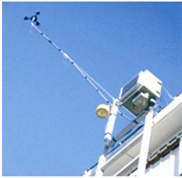
Figure 1. Local meteorological station on school building roof
