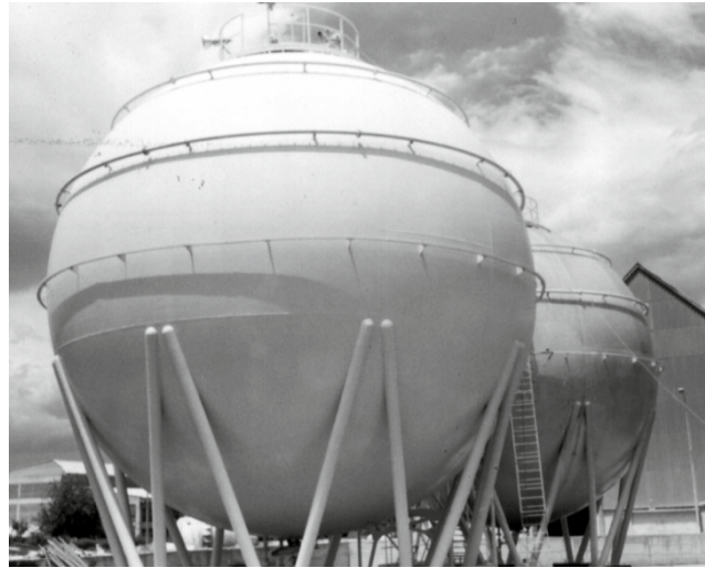
Fig. 3. The spherical tank for ammonia storage
