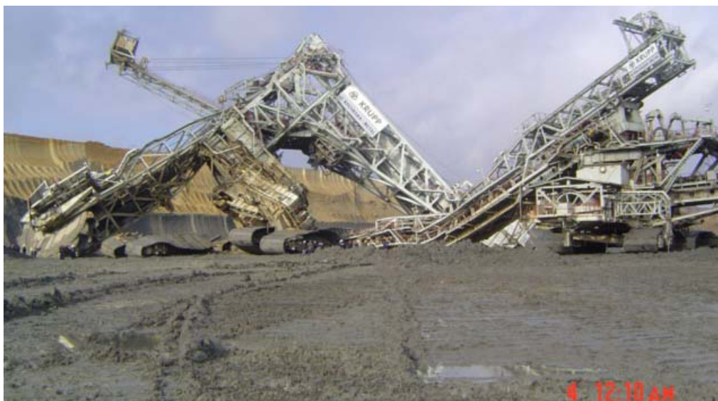
Figure 1. Collapse of bucket wheel excavator SRs 1760.
