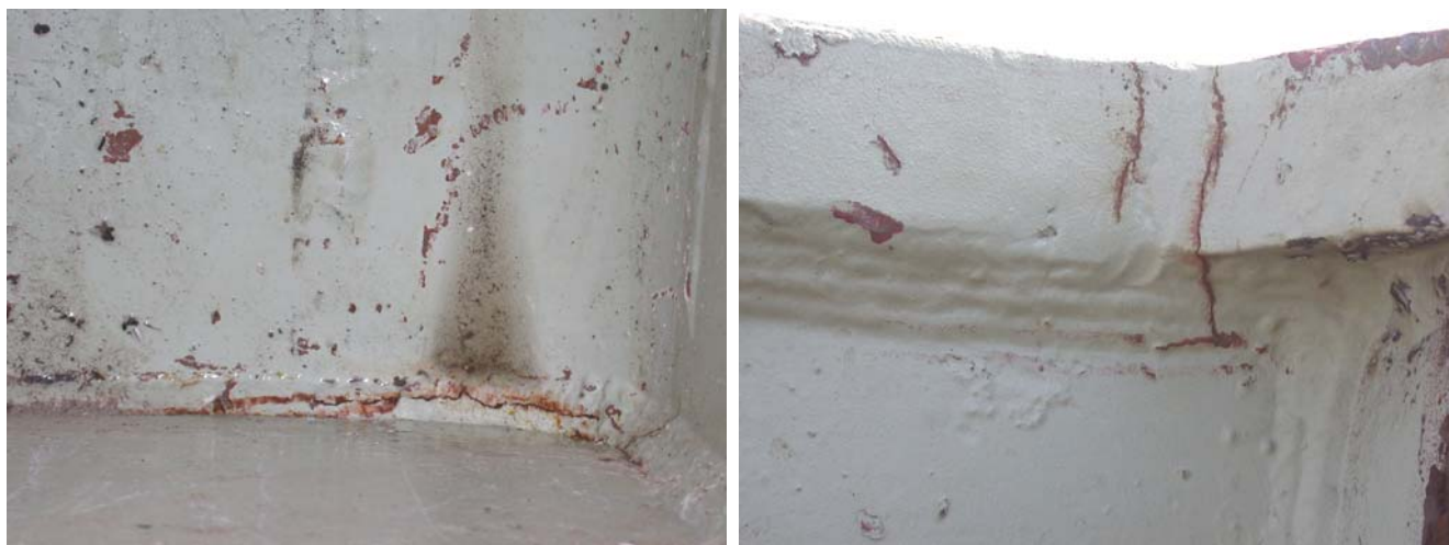
Figure 2. Cracks on the mast of BWE.
