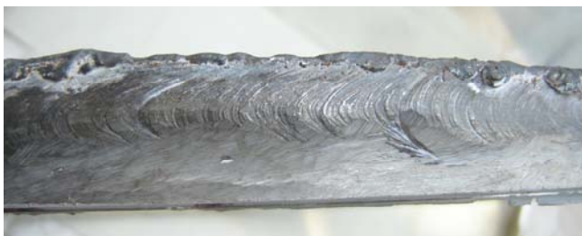
Figure 5. Cylindrical part of the flange and welded joint between the flange and mantle of the manhole.
