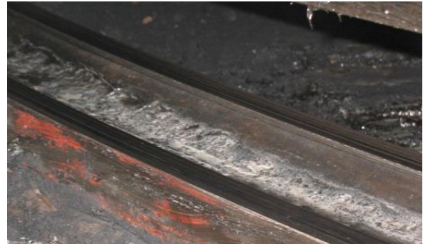
Fig. 15 Wear of bearing upper surface raceway
