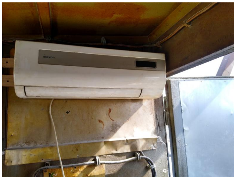
Figure 5. Air circulation based on the use of air conditioning in the excavator cabin.
