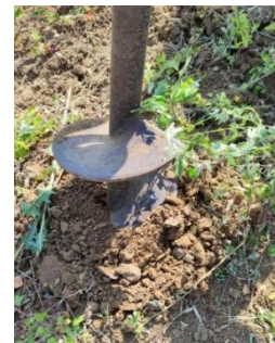
Fig. 3 The drilling process
