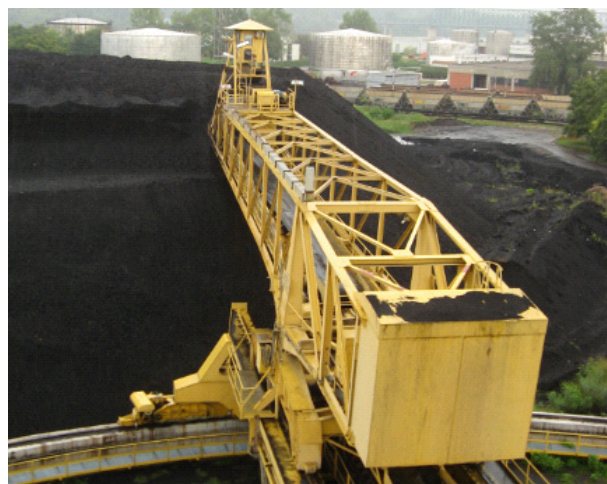
c) Appearance of the bucket-wheel reclaimer (view from behind)
