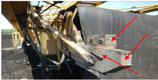
a) Damage that occurred on the carrying structure of the drum (right side);
