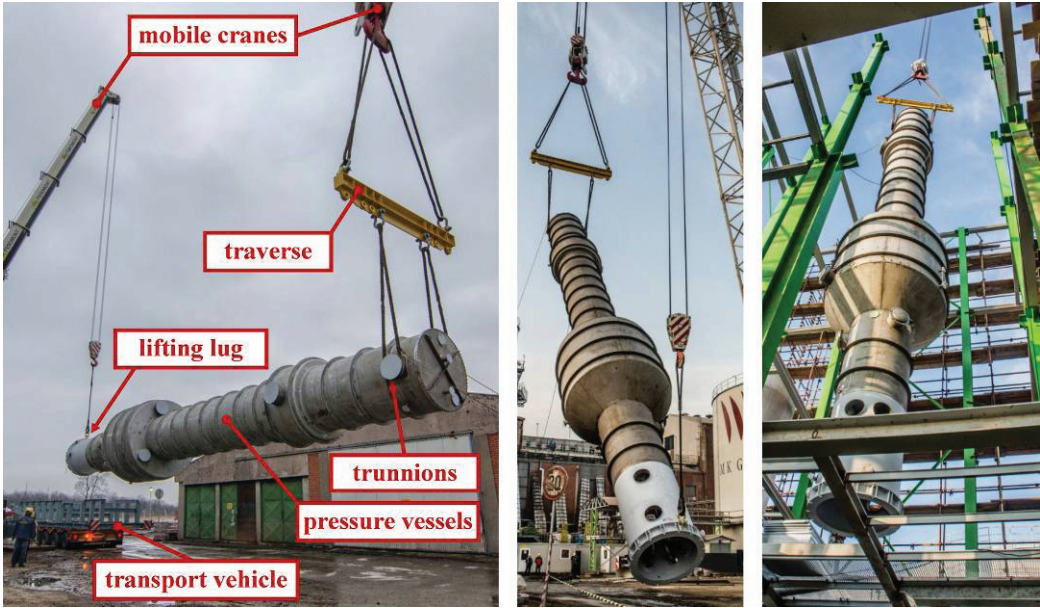
Figure 5: Phases of pressure vessel lifting and positioning
