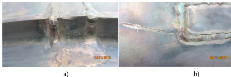
Fig. 6. (a) Crack initiation; (b) Crack propagation from weld into a base material.
