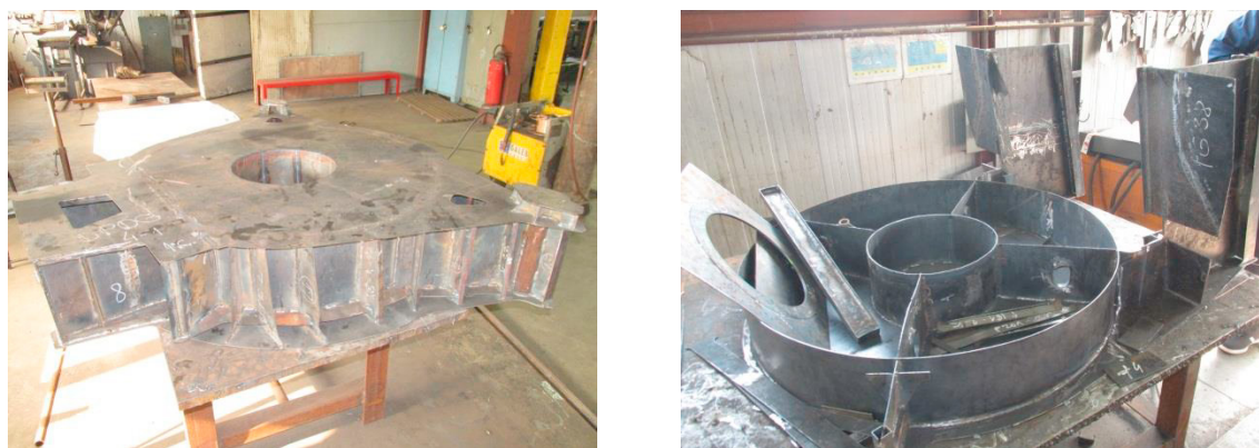
Fig. 1. Substructure (left) and slewing platform with pylons (right) under construction
