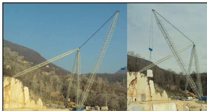
Figure 16: The derrick crane
