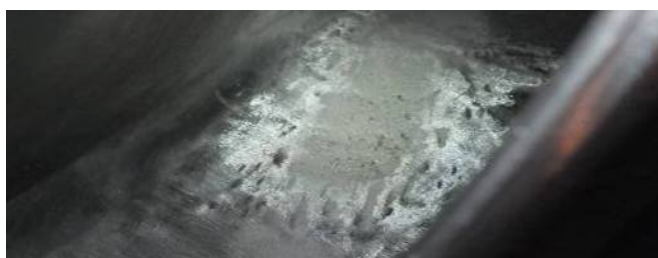
a) cavitation damage on a runner blade
