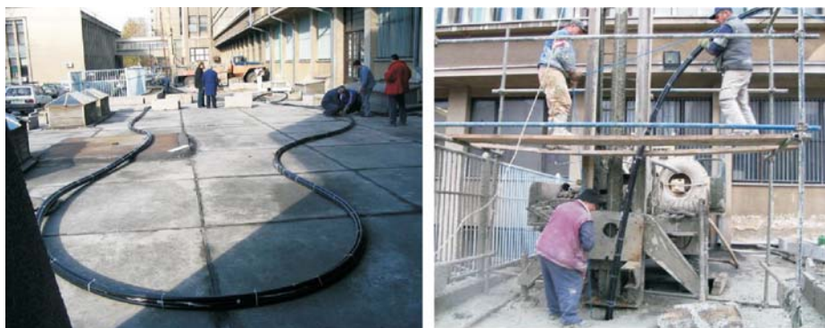
Figure 1. Insertion of the heat exchanger in the vertical borehole
