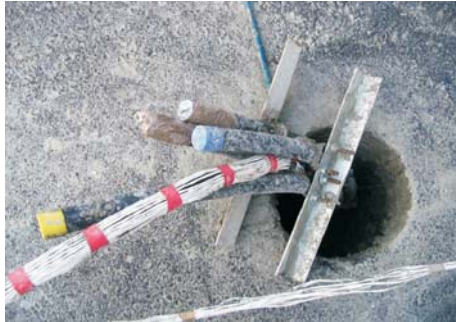
Figure 2. Upper end of (VBHE) before filled by bentonite
