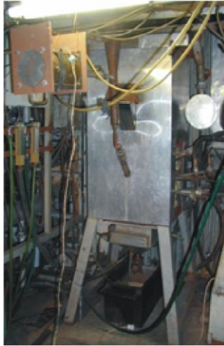
Figure 2. The experimental FB furnace
