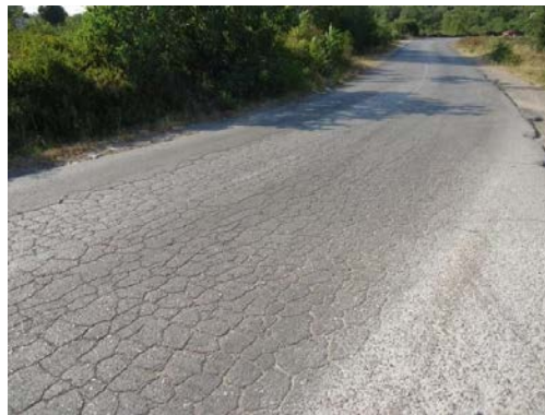
Fig. 5. Asphalt roads built 30–40 years ago.
