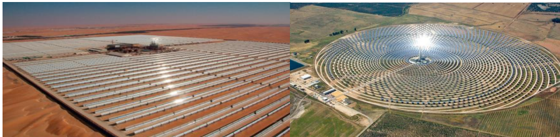
Figure 1. Photovoltaic power plants: "Shams 1" in the UAE (left) and "Ivanpah" in California (right)
