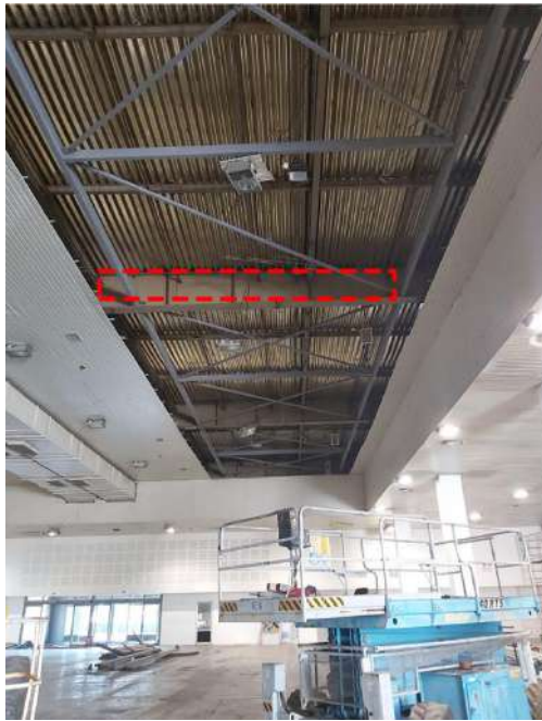
Fig. 1. Roof structure in the attic space
